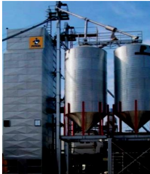
Fig. 4. Dryer with silo cells
