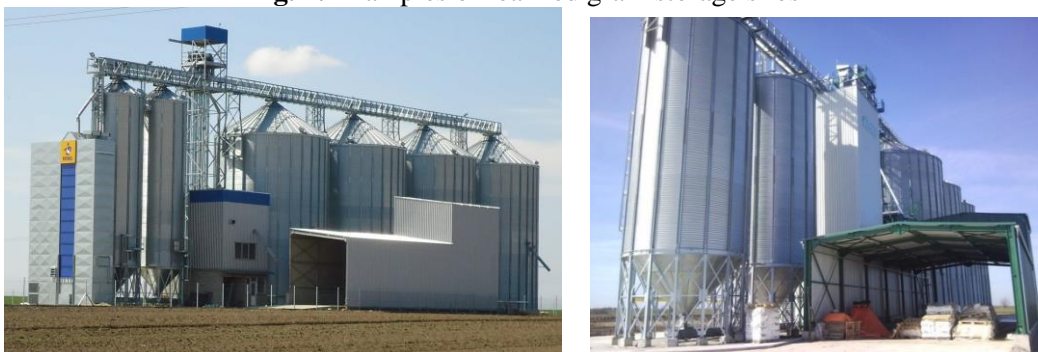
Fig. 3. Examples of realized grain storage silos (silos with a capacity of 5000 t of wheat, transport capacity of 60 t/h), Dryer capacity 18 t of grain 24/14% moisture.
