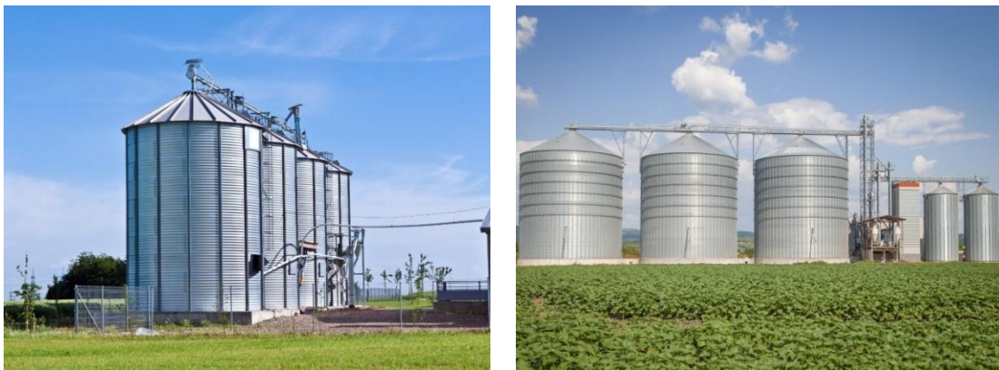
Fig. 2. Examples of realized grain storage silos
